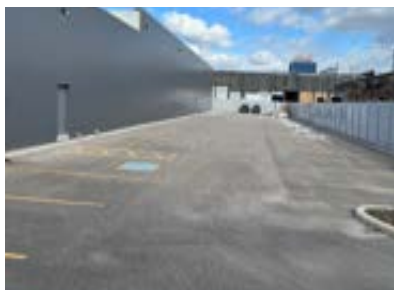
Near Kipling/Evans Studios Parking - Etobicoke 1460 Queensway
